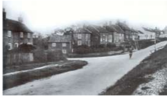
York Road junction showing Primitive Chapel
